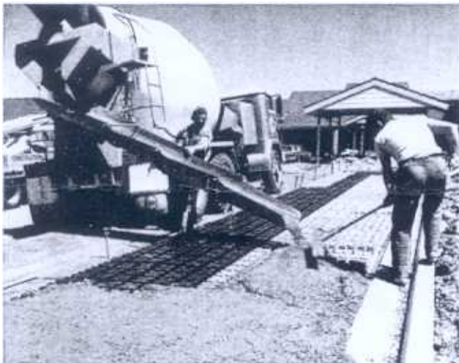
Concrete pouring, and screeding level with the former tops.
